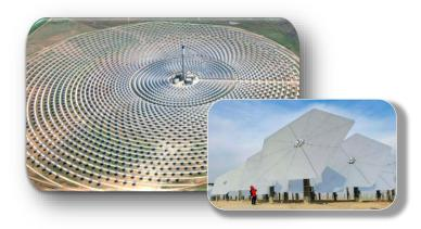
Project:CSP\_SOLAR THERMOELECTRIC 50 MW POWER PLANTTechnology:STELLIO\_HELIOSTAT TECHNOLOGYScope:Electric\_Electronic\_Communications\_Software.Location:China
